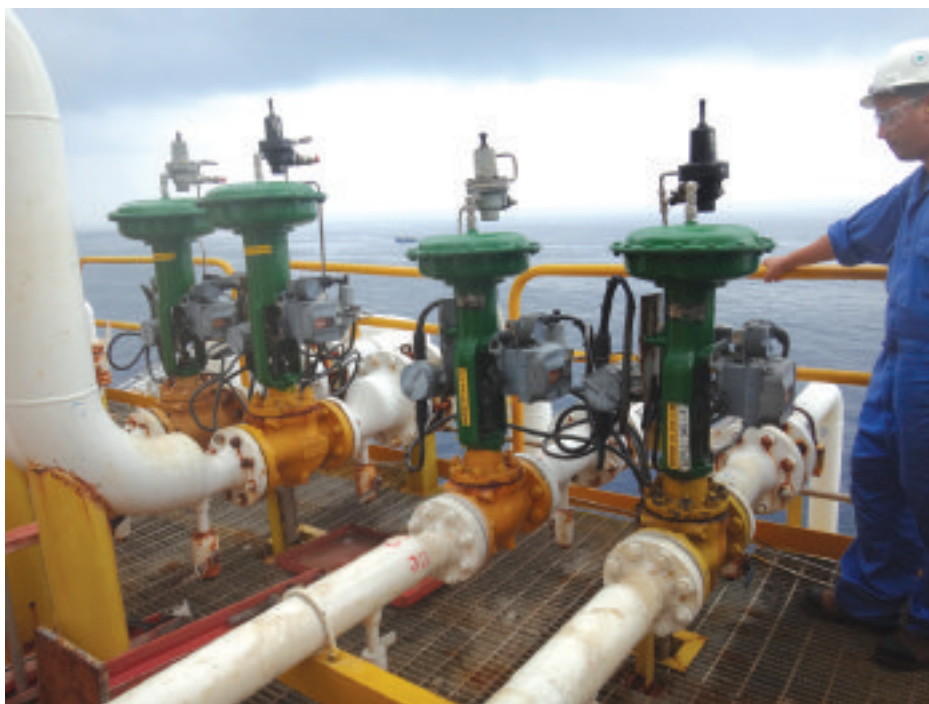
Maintenance of critical components like control valves can go a long way in ensuring process optimisation and uptime. Courtesy: Intech Process Automation
