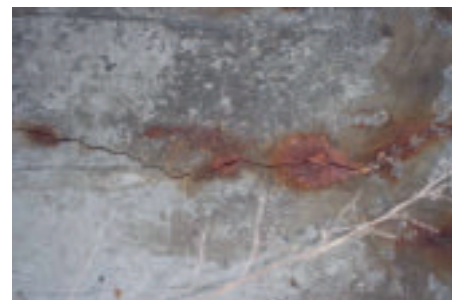
Figure 2: The beginnings of the oxidation process in a pylon of an overpass structure.
