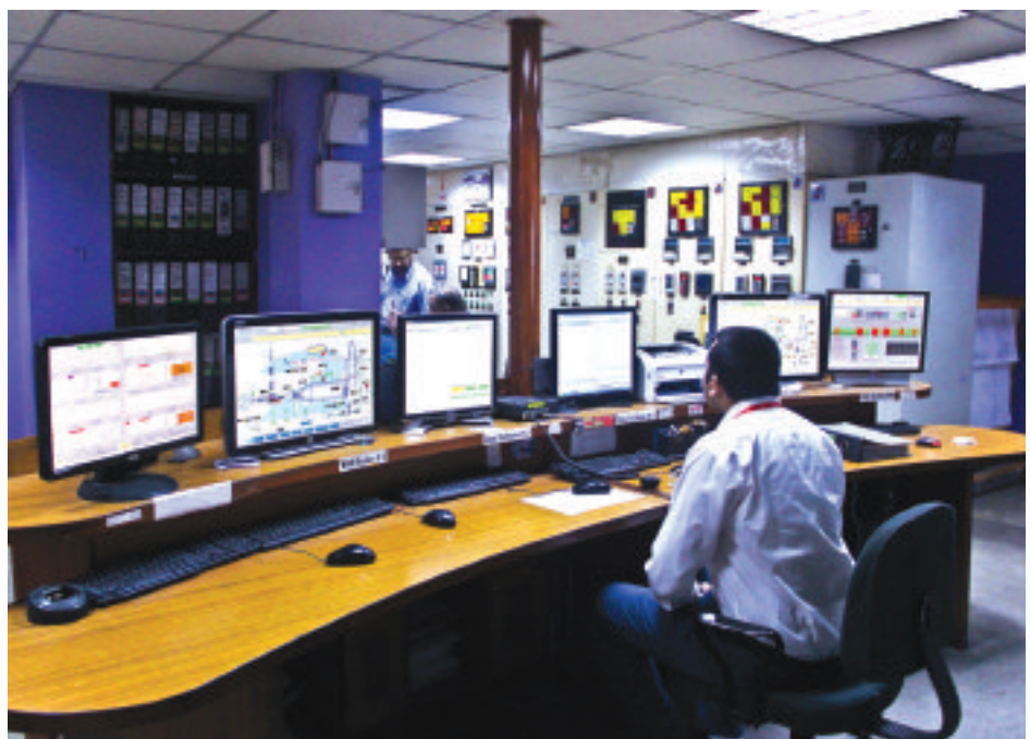
Well-trained operators and a distraction-free control rooms can ensure prolonged uptime of midstream facilities and prevent significant incidents. Courtesy: Intech Process Automation
