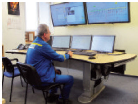
An Inelsev operator overlooking power distribution at the ethylene plant.
